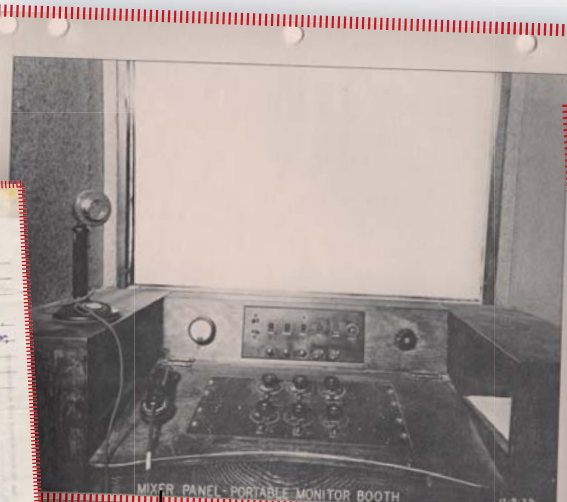
Typical portable monitor booth as used on stage. (From Western Electric/ERPI Manual ca. 1930)
