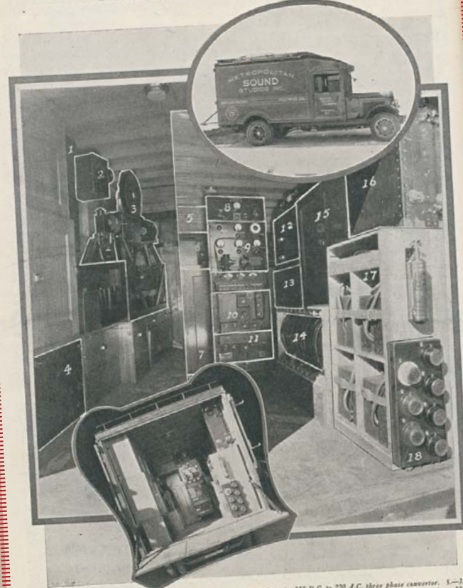
1—Recording panel. 2—Start and control console. 3—Film recorder. 4—110 D.C. to 220 A.C. three phase converter. 5—150 watt dry D.C. 6—Synchronizing motor. 7—Storage battery compartment 110 D.C. 8—Gain set. 9—Oscillator motor. 10—wall dry D.C. 11—27 "8" Amplifier. 12—Charging control panel. 13—Synchronizing control. 14—Film recorder magazine. 15—Microphone cabinet. 16—Mixer panel. 17—Camera motor extension. Courtesy of Helmer W. Bergman, Technical sound Expert, Metropolitan Studios.
