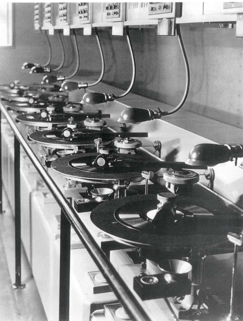
Disc dubbing operations at Warner Bros. Studio circa 1930 (Courtesy George R. Groves Estate)
